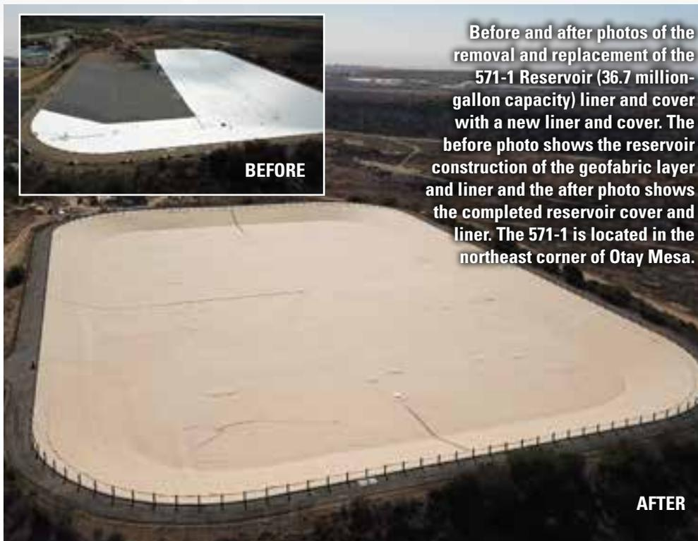
Before and after photos of the removal and replacement of the 571-1 Reservoir (36.7 million-gallon capacity) liner and cover with a new liner and cover. The before photo shows the reservoir construction of the geofabric layer and liner and the after photo shows the completed reservoir cover and liner. The 571-1 is located in the northeast corner of Otay Mesa.
